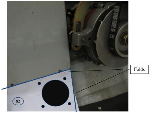
Drill 4 holes diameter 5mm in the aluminium sheet.
